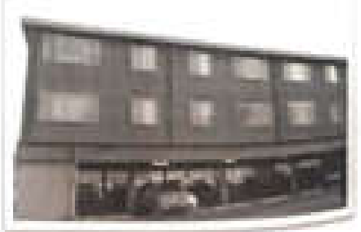
Fig. 1. Typical provision for Open Ground Storey
